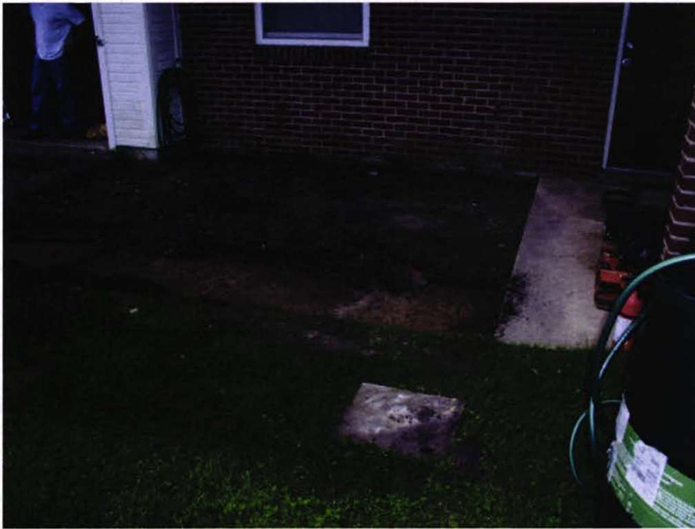
137 Laurel Bay Blvd- Prior to excavation
