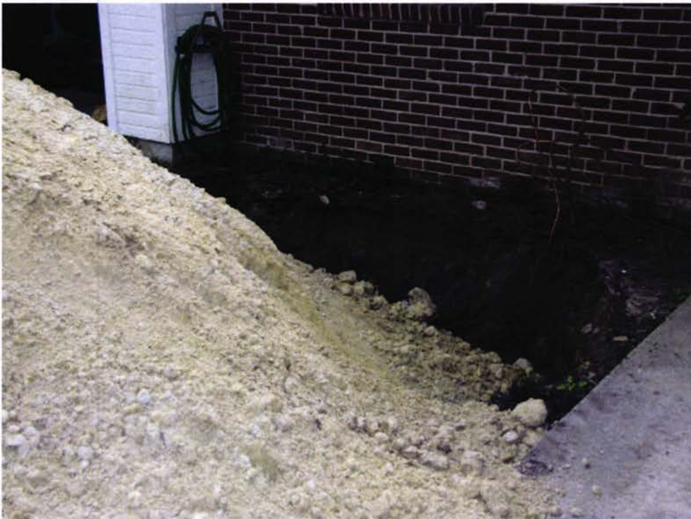
137 Laurel Bay Blvd- Backfill material
