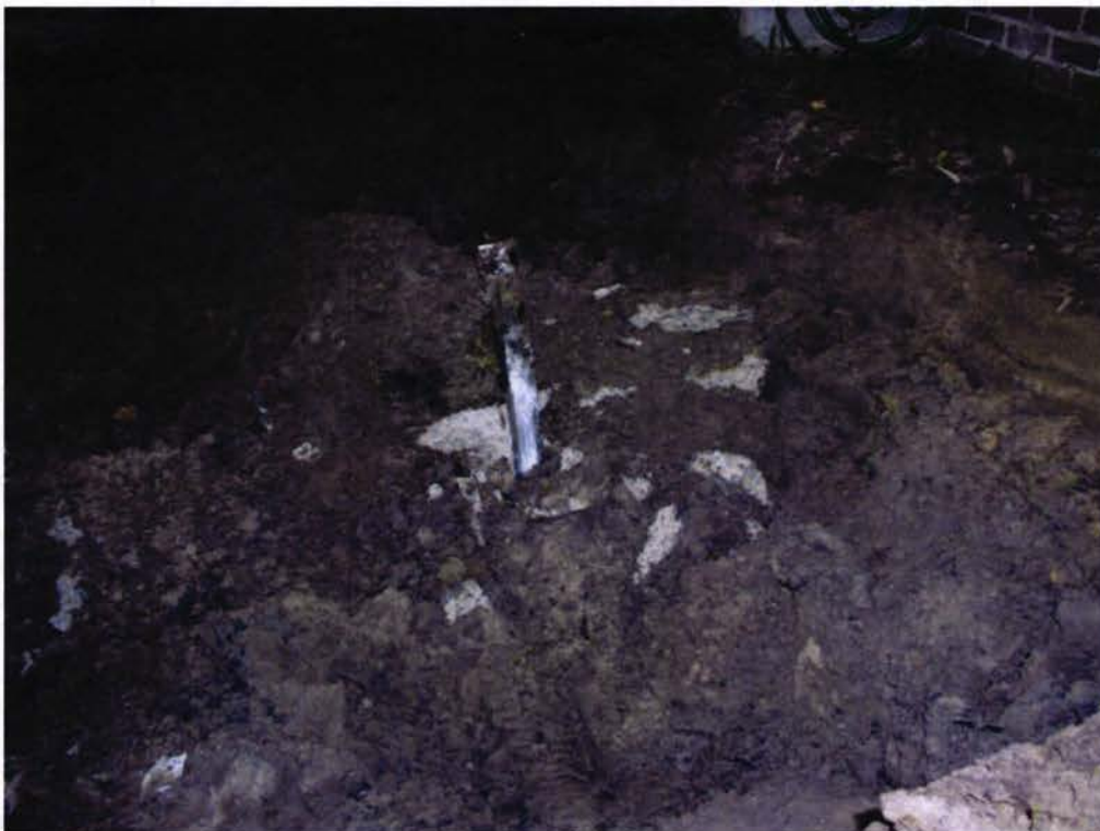
137 Laurel Bay Blvd-Top of Tank
