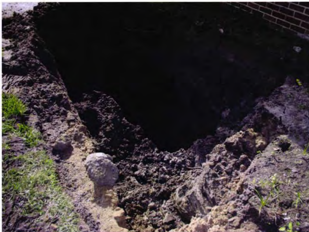
137 Laurel Bay Blvd-Excavation
