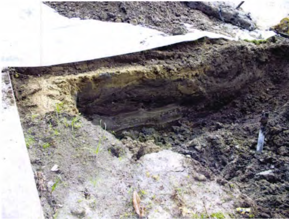
137 Laurel bay Blvd-Excavation
