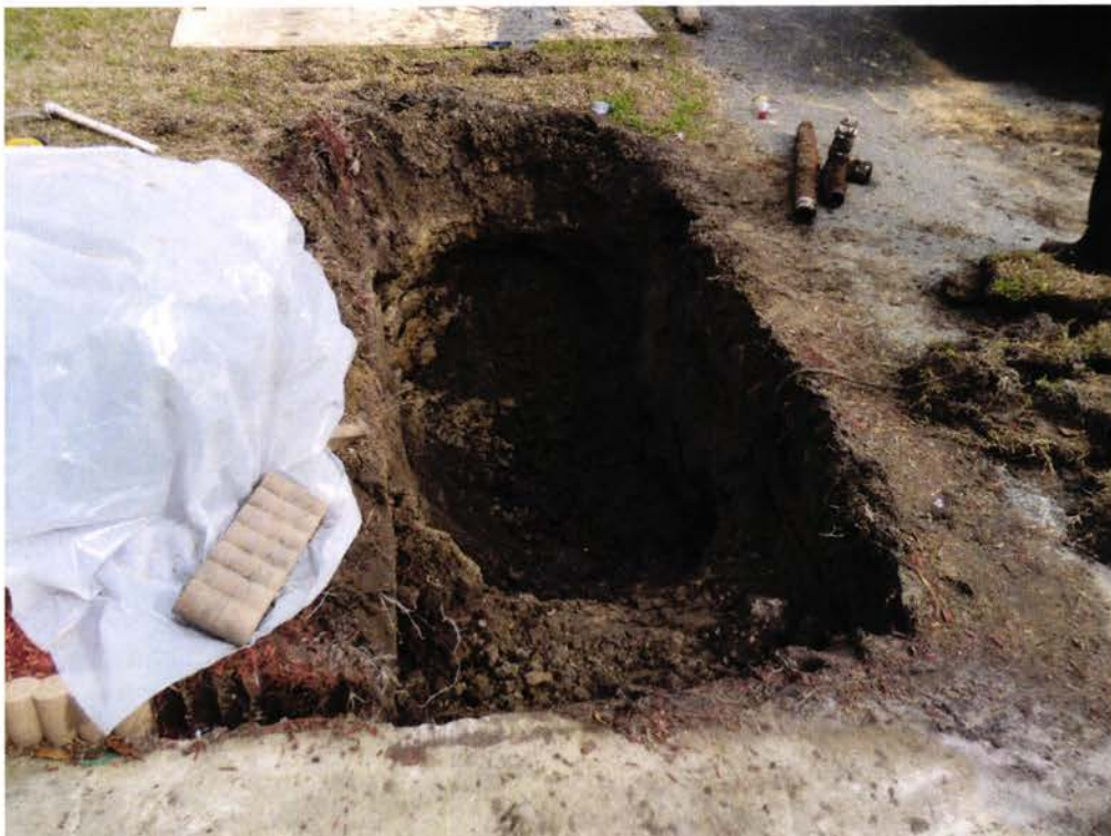
Picture 2: UST 137LaurelBay excavation.
