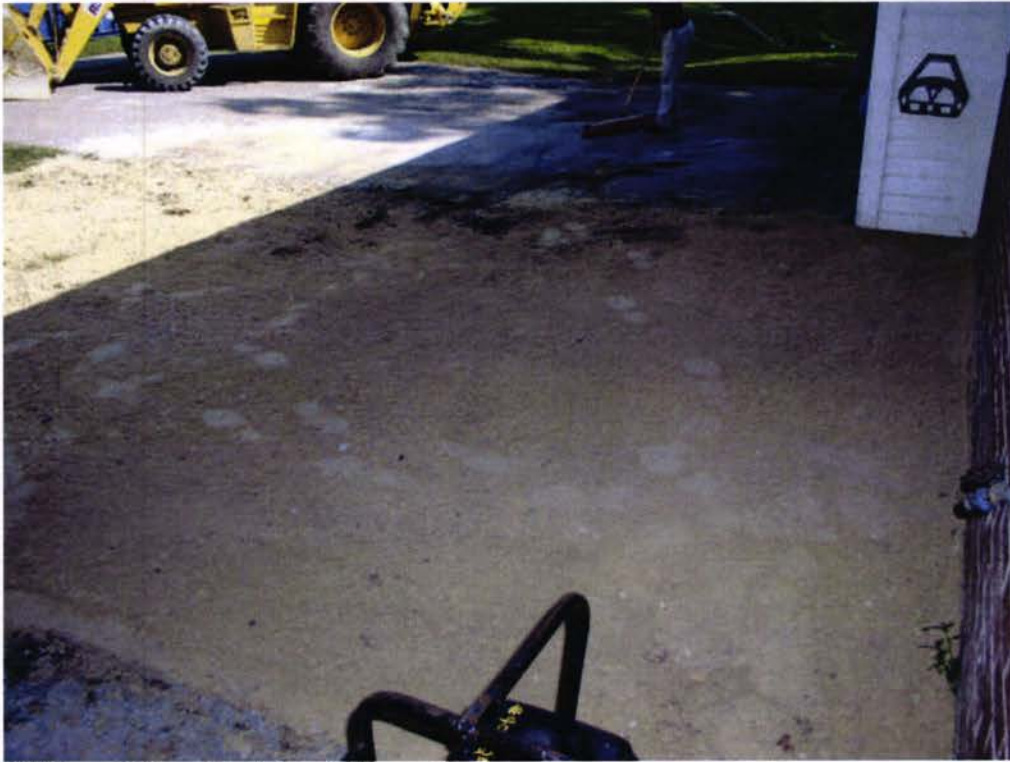
137 Laurel Bay Blvd- Post Excavation
